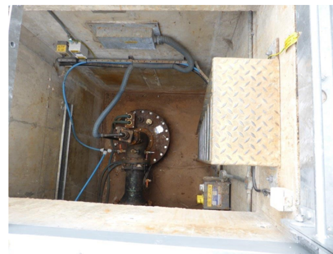
Figure 4 Below ground headworks
