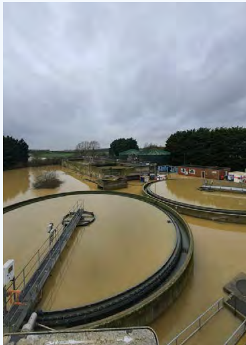
Anwick Water Recycling Centre under water, the source of one of our Category 2 pollutions.
