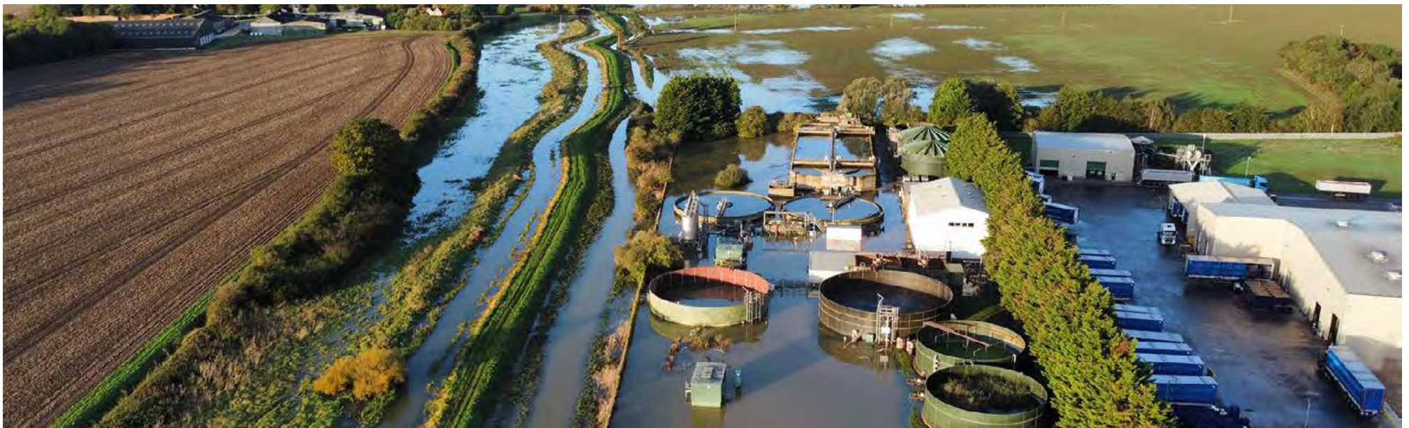
Anwick Water Recycling Centre under water.
