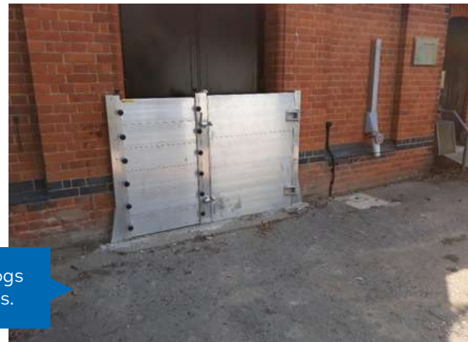
J-Bar flood barrier around critical equipment with swinging barrier at Gosfield Water Recycling Centre
