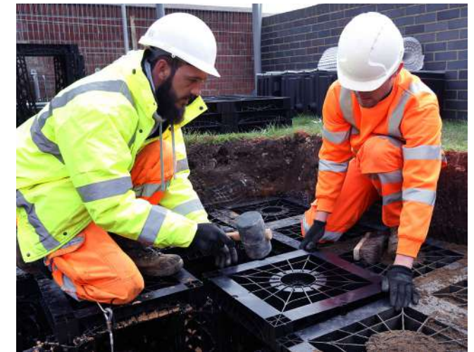
SuDS installation at a school in Newmarket as part of the Make Rain Happy campaign
