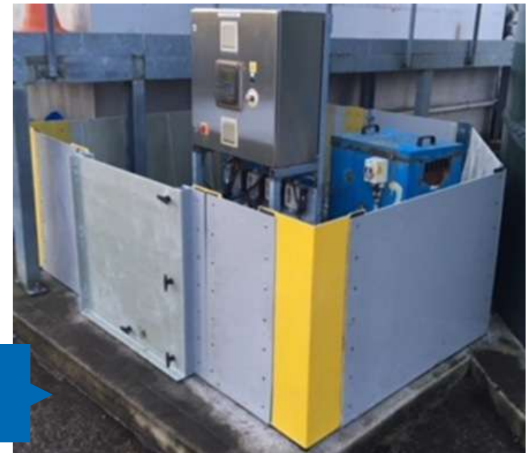
J-Bar flood barrier around critical equipment with swinging barrier at Gosfield Water Recycling Centre
