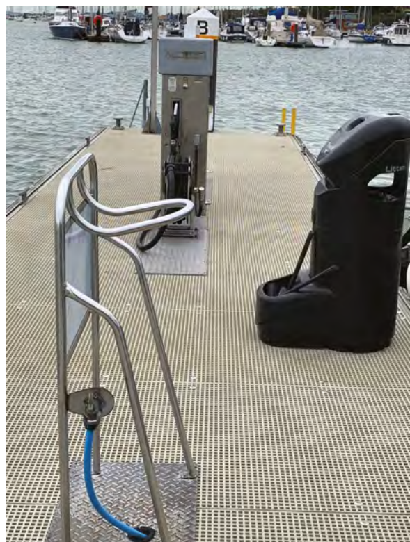
D. Fuel dock with HUT for hose use
