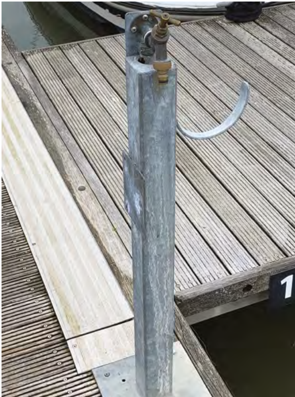
A. Hose union tap on secure pedestal
